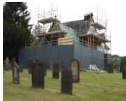
All Saints Dale Abbey Restoration in progress
